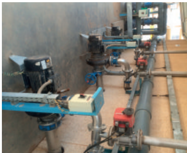
The AirJet propeller-aerators from Landia handle aeration, anoxic tanks and sewage prior to Dissolved Air Flotation (DAF).
